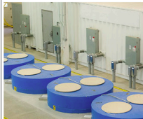
Flywheel Schwungrad storage a 20MW provide
